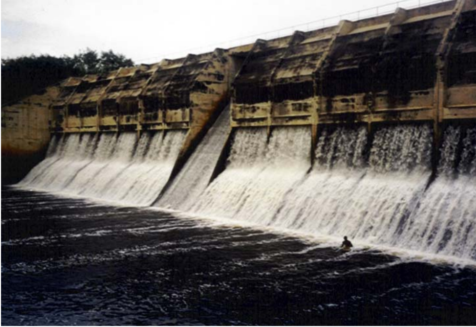
Photo 12: Barekese Dam in Rainy Season
