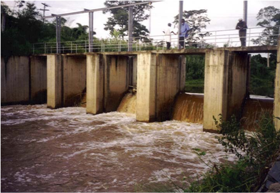
Photo 8: GWC Headworks at Hohoe, Dayi River
