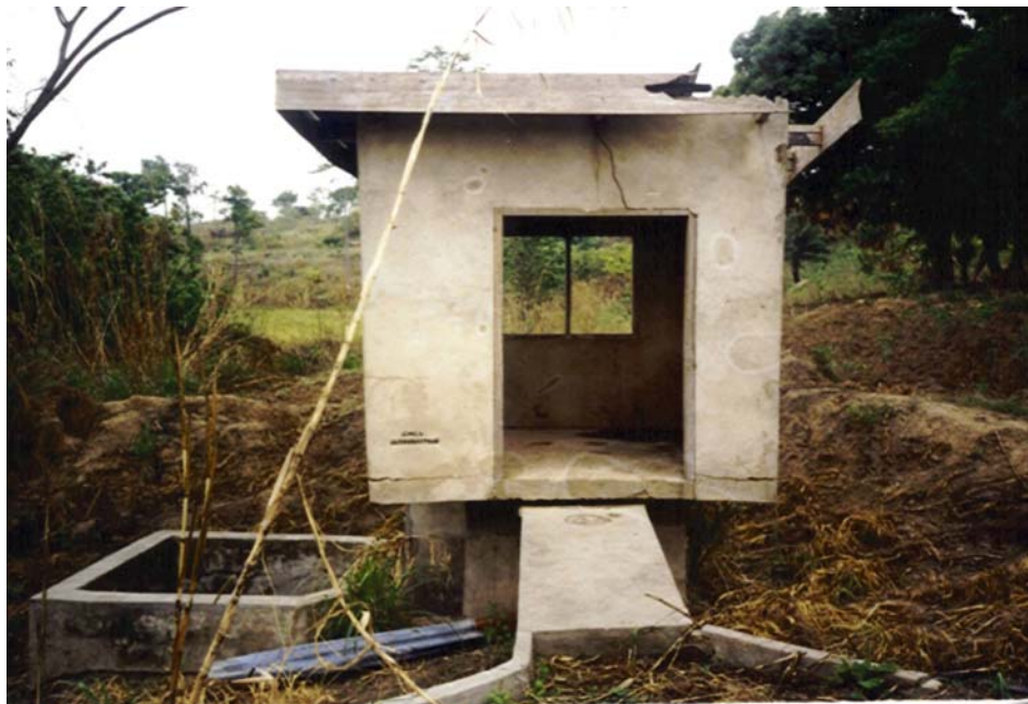
Photo 13: A GWC Pumping Station on Fia River at the site. It has never been in operation
